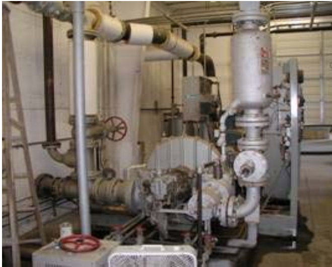
500 kWe Back Pressure Turbine NH
