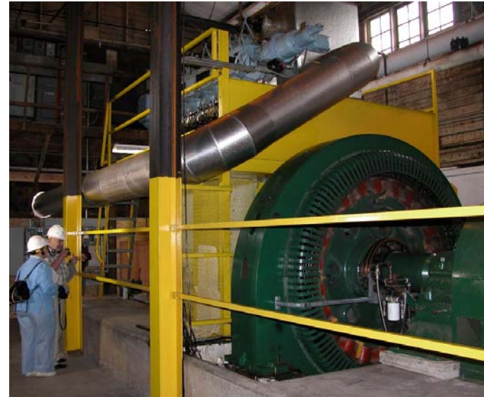
800 kWe 1930s Skinner Steam Engine, WA (No recent US steam engine installations)
